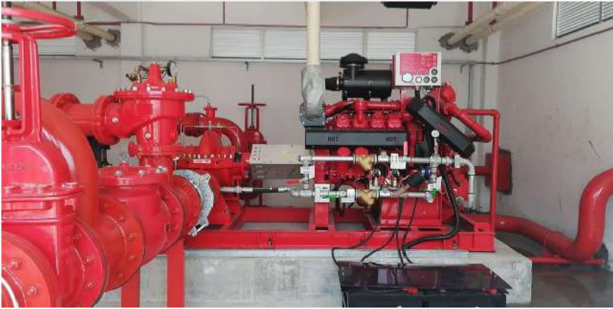
Project: Oil Terminal Fire Fighting Pump (Shell Philippines)
